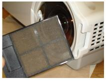
Examine filter for dust particles or dirt blockage
